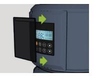
Fit UV Screen cover to the control panel using a strip of d/sided tape across top edge
