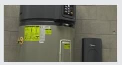
If the controller is indicating an E0 error, then there is an issue with the upper tank sensor. To access the tank sensors, start by removing the front fascia at the front of the unit. Simply grip the fascia from either side and firmly pull the whole piece away from the tank to release the three holding magnets from the tank body. Then put the fascia aside.
