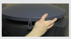
Start by removing the rain shield (where applicable) by removing the fasteners at the four tab locations and then lifting the shield up and putting aside.
