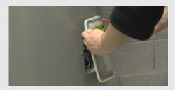
If the controller is indicating an EE error, then there is an issue with the circuit of the E-heater To assess this error, proceed to access the element compartment located in the lower compartment under the front fascia cover. Remove the lower electrical cover by removing the array of screws and put cover and fasteners aside.
