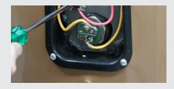
With power activated to the unit, carefully test the element is receiving 240 Volts with a multimeter by placing each of the prongs on the two terminals. If 240 volts is evident then there appears to be an issue with the element. If this is the case isolate power to unit and proceed to replace the element.
