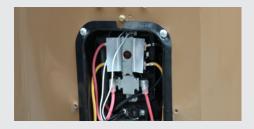
If 240 volts is not evident, we need to test all the corresponding connections back to the PCB to locate where the error exists. Proceed to carefully test the thermostat. If the thermostat is showing 240 volt supply, then the issue lies between the automatic thermostat and the element. If the automatic thermostat shows no voltage then continue to test up the line for correct voltage.
