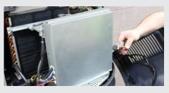
Once the screws are removed carefully pull the front casing away enough to access the controller connector and release. Then put the front casing aside.
