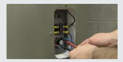
If the manual thermostat has not been tripped, then we need to proceed to test the automatic thermostat for 240 volt supply. Again with power activated to the unit, carefully test the automatic thermostat. If the automatic thermostat is showing 240 volt supply, then the issue lies between the automatic thermostat and the element. If the automatic thermostat shows no voltage then continue to test up the line, checking the manual thermostat for correct voltage.
