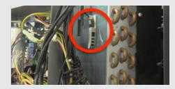
The Ambient Temperature sensor is located on the right hand side fitted to the face of the evaporator.
