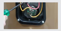
With power activated to the unit, carefully test the element is receiving 240 Volts with a multimeter by placing each of the prongs on the two terminals.
