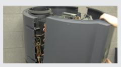
If the controller is indicating an E9 error code, then there is an issue with the Compressor Suction Temperature Sensor (TH Sensor).
