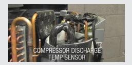
If the parameters on screen confirm there is a difference of less than 10 degrees, then we need to perform a manual check, testing the temperature of each location. If the manual readings support both of the on screen readings then it would appear that there is a compressor issue. If one or both manual readings are significantly different then the corresponding sensor may need to be replaced. (Refer to the relevant instruction)
