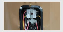
If 240 volts is not evident, we need to test all the corresponding connections back to the PCB to locate where the error exists. Proceed to carefully test the thermostat. If the thermostat is showing 240 volt supply, then the issue lies between the thermostat and the element. If the thermostat shows no voltage then continue to test up the line for correct voltage.
