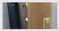
If the controller is indicating an error of E1, then there is an issue with the tank sensor. To access the tank sensors, start by removing the front fascia at the front of the unit. Simply grip the fascia from either side and firmly lift vertically to release the pins at the top and the holding bracket at the bottom, then pull the whole away from the tank body. Then put the fascia aside.
