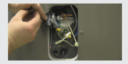
If you are presented with an error code of E0, then this relates to the upper tank sensor (referred to as Sensor T5U).
