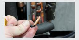
To access the sensor, cut the cable tie. Remove the sensor from its container and inspect for any visual damage and check that the corresponding connector to the PCB board is securely seated.
