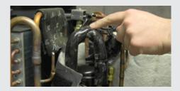
The Compressor Suction Temp Sensor is located on the inlet pipe to the compressor To access we need to remove the insulation of the compressor by removing the two Velcro tabs.
